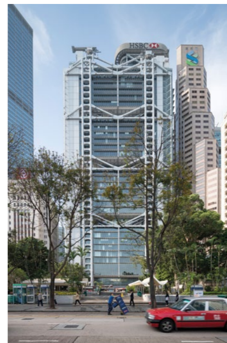
2020 UniFor realises, based on Hassell's design, the interior project for the QRC Suites in the HSBC building in Hong Kong.
